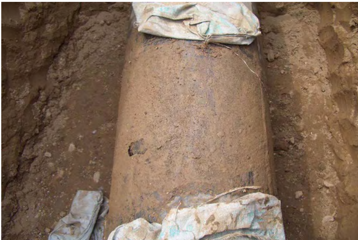
Figure 10 Uncoated Pipeline Joint
