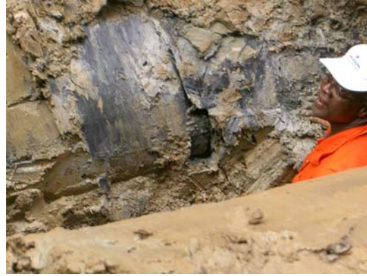
Figure 16 Coating Defect Located by CIPS/DCVG Survey
